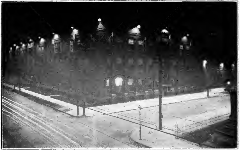
Protective Lighting at the East Forty-fifth Street Plant
